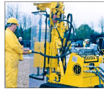
Figure 2. Indicative size of piling rig that may be used
